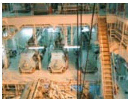
Fig. 4 Three diesel gen-sets in parallel controlled by SIGMA
